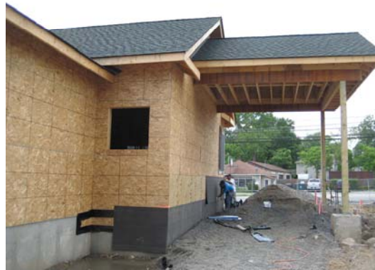
A better view of the drive thru canopy a few weeks later. Laborers hard at work installing the underlay for the stone façade.
